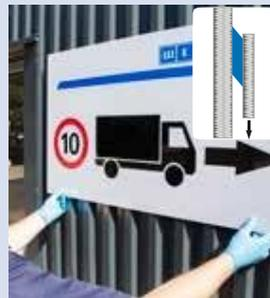
In vertical adhesive bondings, e.g. attaching panelling elements to walls, the bonding is exposed to shear stress. Due to this, the major part of the load should be close to the adhesive surface, so the load does not generate peel or split tensile strength.
