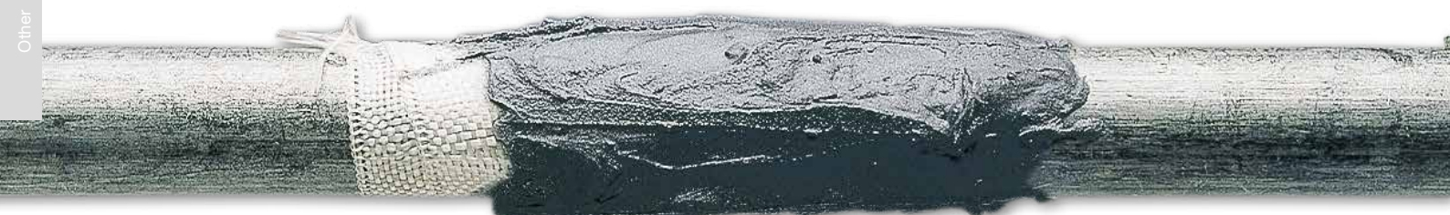
Emergency repair of a water pipe
